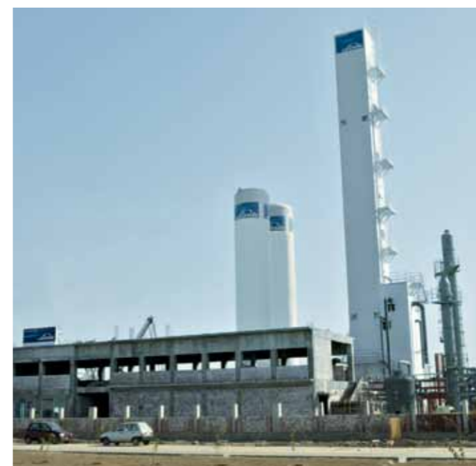
Sundar ASU Plant nearing completion
